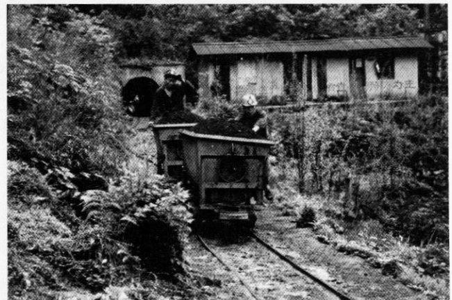
Tubs of coal being manually pushed from Huangchunjing adit at Huangcun Mine. Photo Ken Geddes
